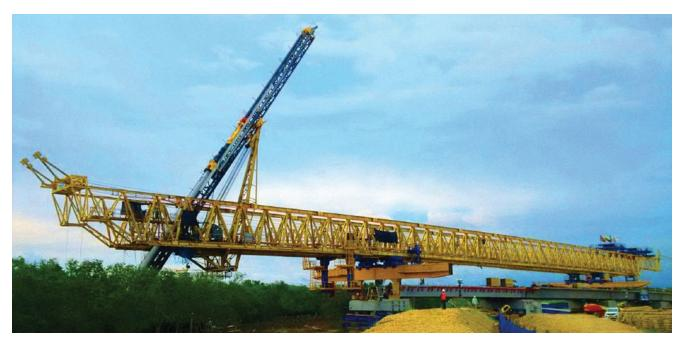
2015, Stefano Gabaldo of Bermingham was contacted by DEAL (of Italy) to assist with the piling portion of a new Beam Launcher project in Cartegena, Colombia. DEAL parent company of Rizzani de Eccher was to build a 5 km bridge with bents spaced at 37 meter increments. This bridge was the final section of the highway connecting Barranquilla to Cartagena to be upgraded.
